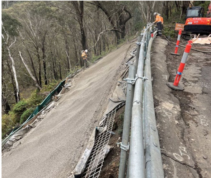
Stabilisation work is being carried out PIC: Transport for NSW
